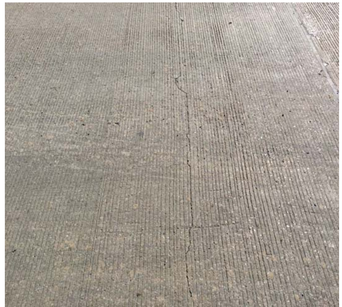
PHOTO 2 Description Approach slab @ Abutment 2 cracking.
