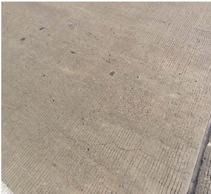
PHOTO 1 Description Unsealed cracks to deck @ all spans.
