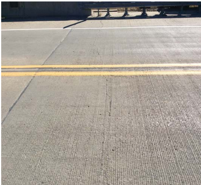
PHOTO 1 Description Approach slabs @ Abutments 1 & 2 have unsealed transverse cracks.
