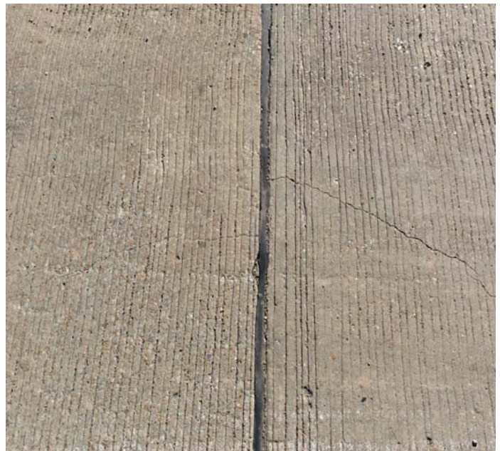
PHOTO 2 Description Unsealed cracks to deck @ all spans.
